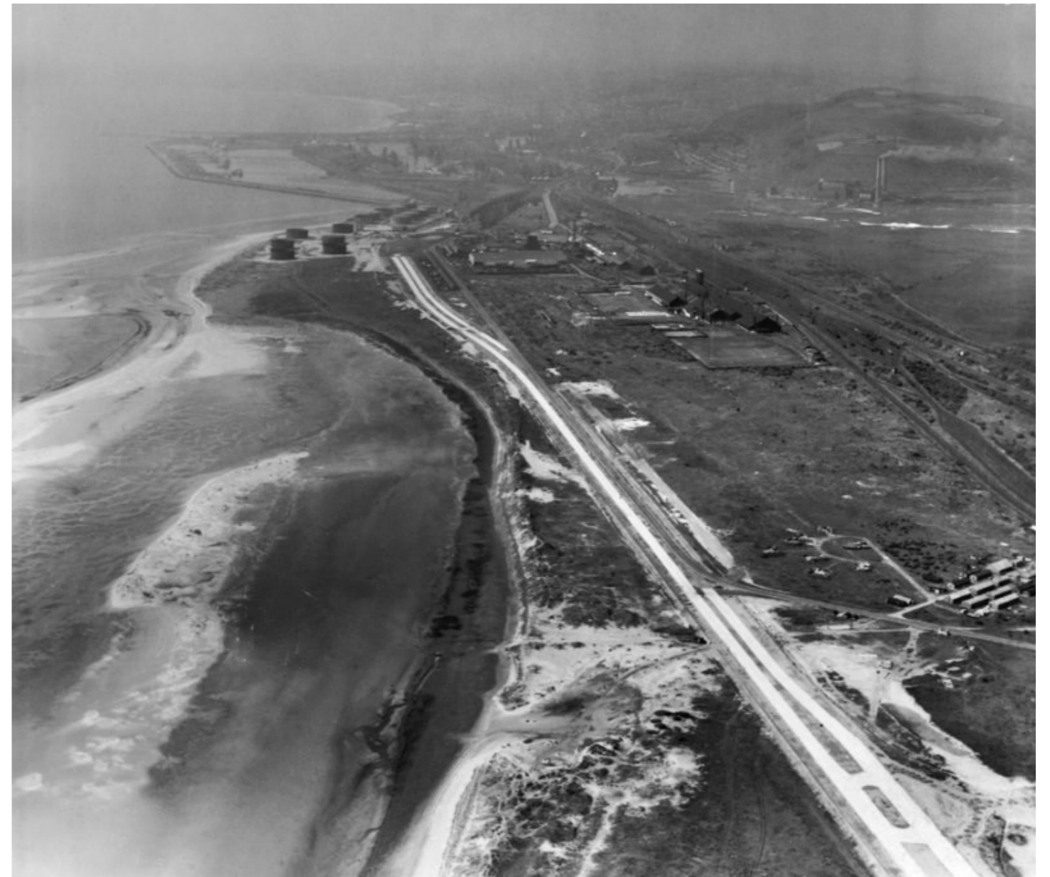
Fabian Way, or Jersey Marine Road, now A483, was constructed between May 1946 and September 1950. Amazon now lies to the right of the dual carriageway and the bay area was reclaimed for petro-chemical tanks, now the Swansea University Bay Campus.
